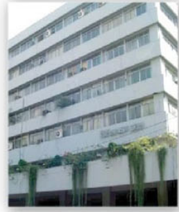
Bangladesh Taar & Telephone Board 500 KVA Substation & Generator
