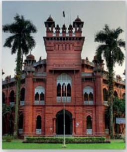
Dhaka University 440 & 330 KVA Generator, Movi Passenger Lift
