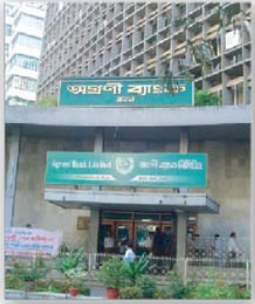
Agrani Bank Ltd. 500 KVA Cummins Generator
