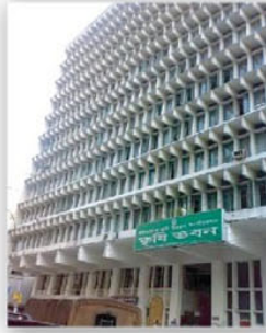
Krishi Bhaban 350 KVA Mercedes-Benz Generator
