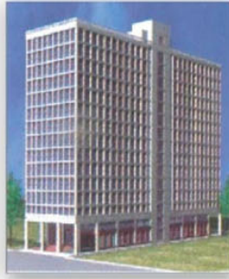
ASA Head Office 770 KVA Denyo Generator
