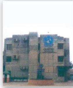
ICDDR Hospital 7 Nos passenger lift & 750 Ton INFINITY Split Type Air Conditioner
